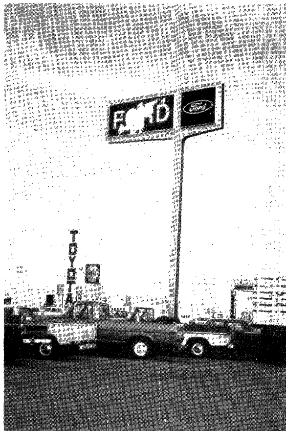
Figure 14. "Ford" sign in Wetaskiwin broken by the hail from the July 6, 1975 storm. Also in the background is the "Action Muffer" sign broken.
